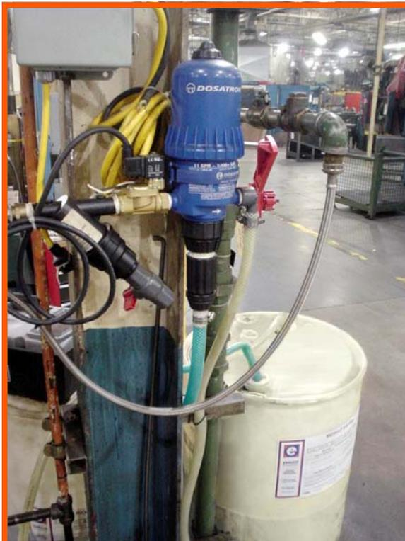
*Dosatron dispensers provide on-demand, consistent coolant dilution, compensating for changes in water pressure and flow.*
